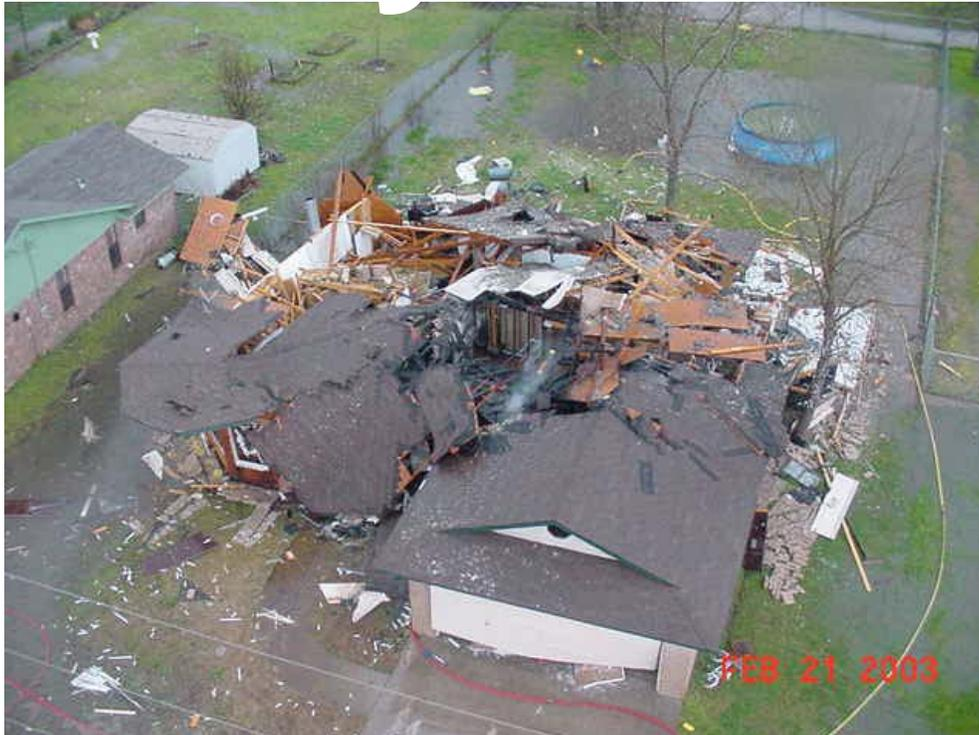
Gas related damage to a home in Texas. This is the type of damage that can result when lightning arcs and travels on CSST
